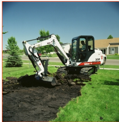
337 Excavator with Grading Bucket
