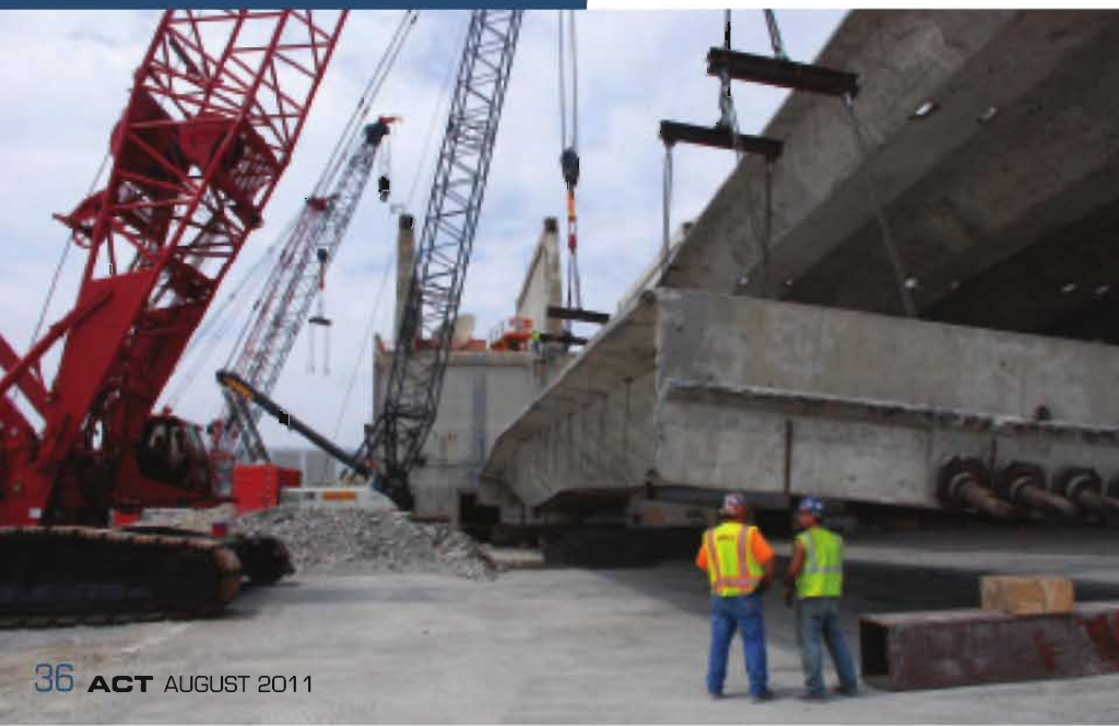
The slabs were 145-foot long, 25-foot wide and weighed 370,000 pounds. There were 56 panels to prepare and lower to the ground. The roof slabs were secured and supported through a load utilization system employing lifting frames, equalizing beams and rolling blocks. Once braced, rigging crews prepared the concrete slabs for sawing and made the final cuts in the rebar that connected the slabs to the core
