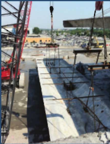
The slabs were 145-foot long, 25-foot wide and weighed 370,000 pounds. There were 56 panels to prepare and lower to the ground. The roof slabs were secured and supported through a load utilization system employing lifting frames, equalizing beams and rolling blocks. Once braced, rigging crews prepared the concrete slabs for sawing and made the final cuts in the rebar that connected the slabs to the core
